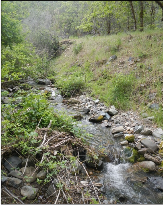
Figure 7. Photograph of the existing alignment of Hotelling Gulch (looking upstream).
