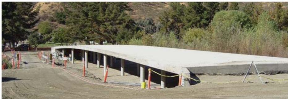
Typical Reinforced Concrete Slab Bridge during Construction
