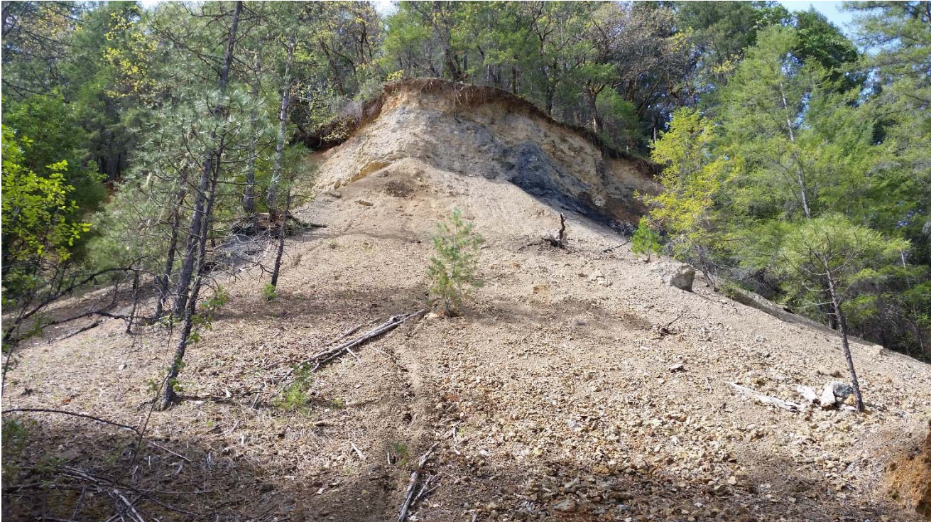
Photo 2. Hydraulically mined hillslope above (south) the HGFCDP area.
