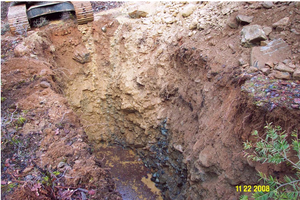
Photo 6. Excavation Test Pit # 7 showing similar stratigraphy.
